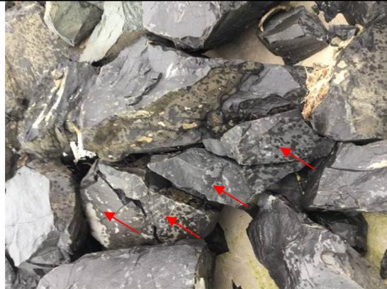
Damage 3 - multiple fractures and residual armourstone likely 750kg or less - #62. Multiple fracture planes
