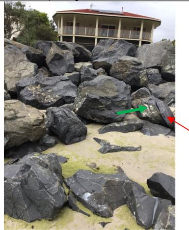
Defect- spalling with main armourstone likely >1t - #74
