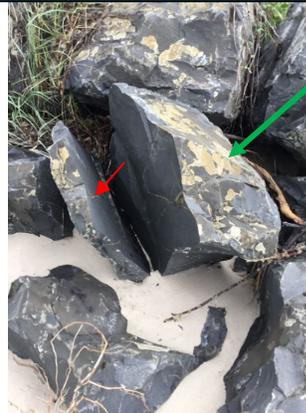
Defect- Spalling with main armourstone likely >1t - #78
