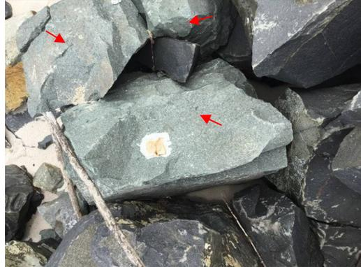
Damage 1 on Marking Plate 48- multiple fractures and residual armourstone likely 750kg or less - Damaged since November 2015. The armourstone seems not to be originating from Dundorwan Quarry - #58. Appears to be a mechanical fracture
