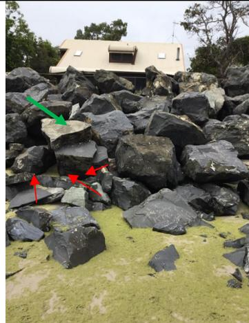
Defect- Spalling with main armourstone likely >>1t - #76
