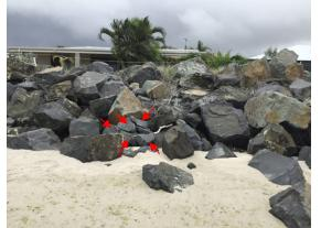
Damage 6 - multiple fractures and residual armourstone likely 750kg or less - #64
