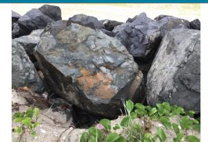
Defect D2: Void at crest due to localised sand slumping Ref No: P12
