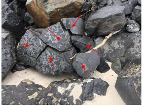
Damage 5 - multiple fractures and residual armourstone likely 400kg or less - #64. Multiple fracture planes
