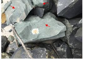
Damage 1 on Marking Plate 48- multiple fractures and residual armourstone likely 750kg or less - Damaged since November 2015. The armourstone seems not to be originating from Dundorwan Quarry - #58. Appears to be a mechanical fracture
