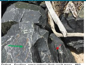
Defect - Spalling, armourstone likely >>1t mass - #50
