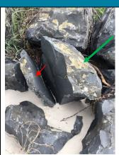
Defect- Spalling with main armourstone likely >1t - #78
