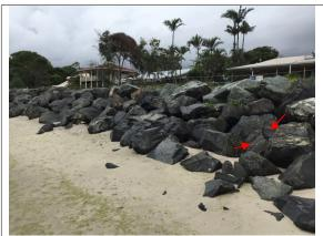
Damage 7 - multiple fractures and residual armourstone likely 750kg or less - #70
