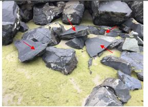
Damage 10 - multiple fractures plane and residual armourstone likely 100kg or less - #76
