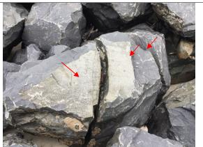
Damage 8 – 3x fractures main armourstone likely ~ 750kg or less #70
