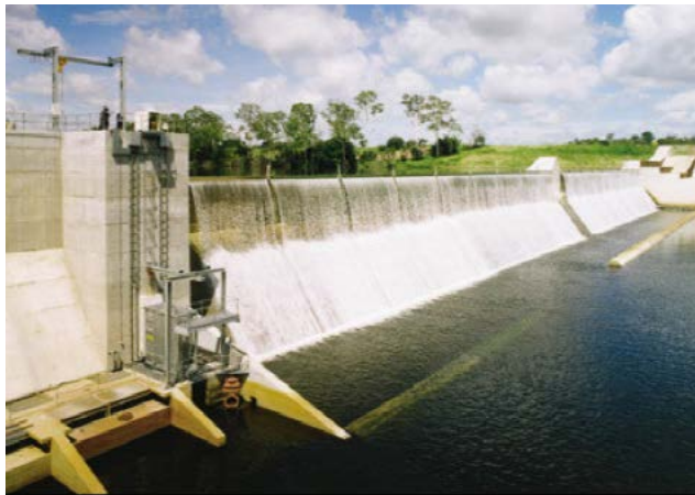
Figure 4.4 Ned Churchward Weir
