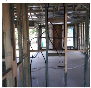
When pipes are concealed in conduit below the floor for island benches, all pipes are to have elbows before entering and after existing the conduit and tails have appropriate fittings fastened to floor in an approved manner.
