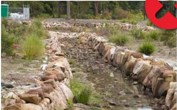
Rock lined trapezoidal channels - poor ecological function, prone to weed infestations, difficult to maintain without using herbicides in waterway
