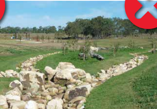
Dumped rock - poor ecological function, prone to weed infestations, difficult to maintain without using herbicides in waterway
