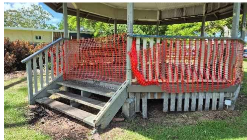
Figure 19: View to side and stairs.
