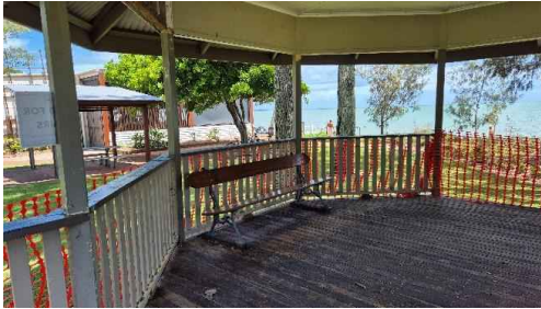
Figure 24: Interior – view northwest.
