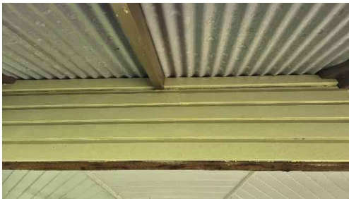
Figure 28: Close-up of exterior of upper section.
