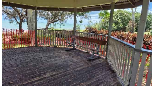
Figure 25: Interior – view northeast.
