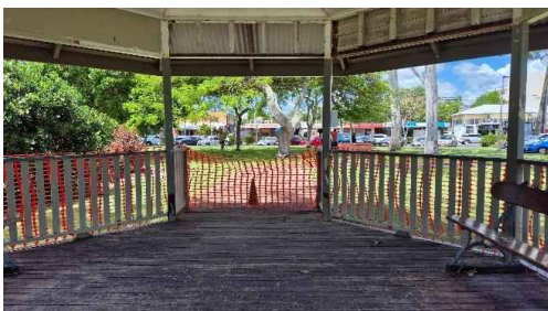
Figure 22: Interior – view to south.
