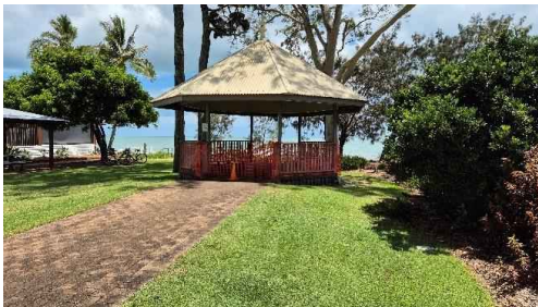
Figure 16: View north to rotunda.
