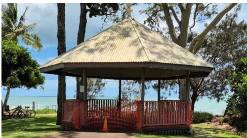
Figure 20: Barrier free access from the south.
