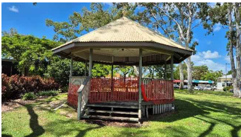
Figure 18: Access via stairs from the north.
