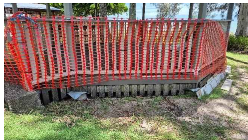
Figure 21: View to side showing concealed undercroft.
