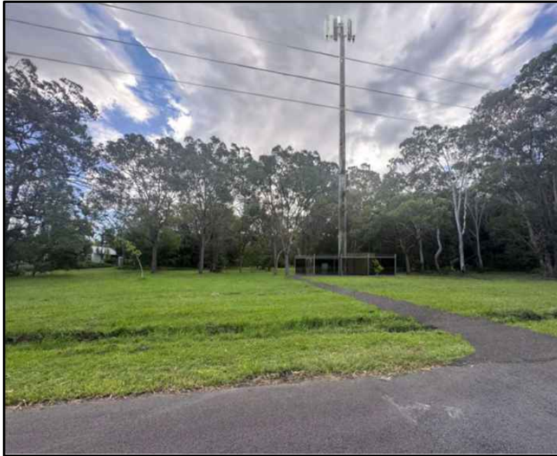
Figure 3 - Location 1 - View from Petersen Road viewing directly at the proposed location of the facility compound
